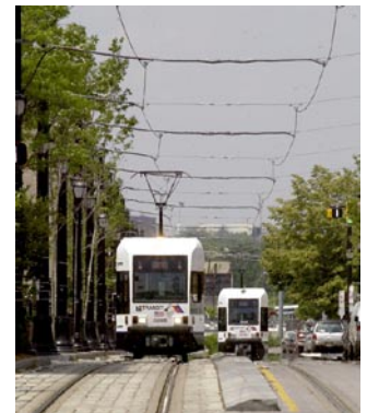
Figures 3 and 4 – At left is an example of a visually unobtrusive single contact wire (ETB) streetcar system in Portland, OR. The photo at right is of Essex Street in Jersey City, where the Hudson Bergen Light Rail line runs in two directions. It is a single wire OCS (cross cabling is support wire to reduce sagging). It also shows the dedicated Light Rail Vehicle lane at left; the right lane is mixed use traffic.
