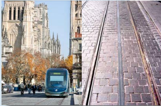
The Bordeaux, France tram system applies an innovative traction power system developed by INNORAIL that replaces the overhead contact system with a power supply imbedded in pavement. Pedestrians can walk on the contact rail, as it is energized only when the tram vehicle passes over it. Vehicle is shown on left and traction power rail imbedded in cobblestone is shown on right. Reliability of the system has not yet been proven.
