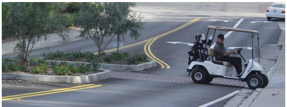
Fore! Median Crossing: median with pedestrian/golf cart refuge, located adjacent to a golf course
