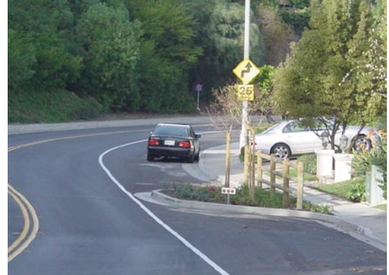
Road narrowing through striping and choker - striping delineation and choker serve to narrow lanes and allow cars to back out of driveways.
