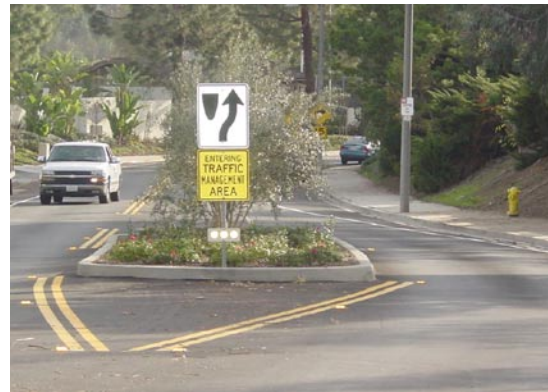
Road-narrowing median with traffic calming signage - entry to traffic calming area. Median narrows the roadway to slow traffic.
