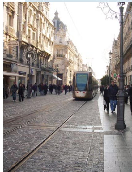
Tram in Orleans, France – typical example of streetscape improvement project in Europe tied to new Tram system project. Catenary wires, attached to the buildings and decorative poles, are barely visible against clear sky. Street was completely redesigned during tram project.
