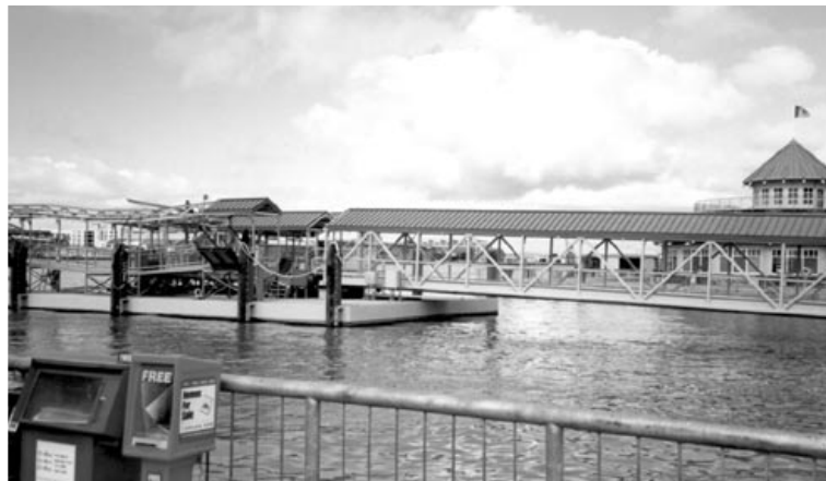
Vallejo, California Ferry Terminal
