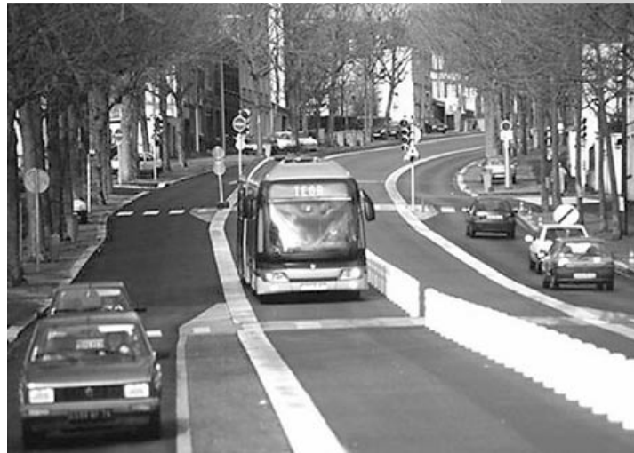
Urban Arterial Median Busway: TEOR System, Rouen, France
