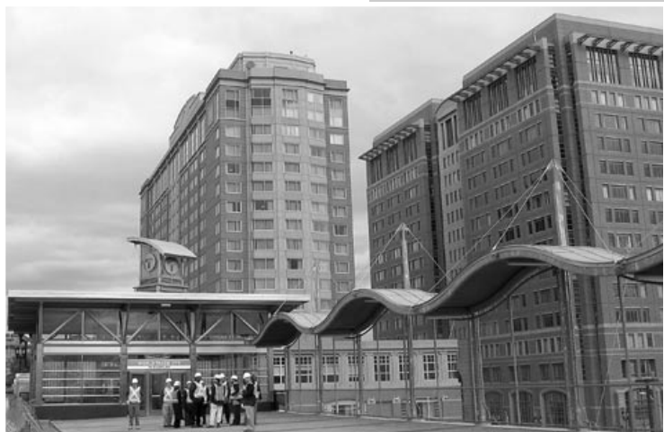
Mixed Use Development Adjacent to Courthouse Station, Silver Line Phase II, Boston, MBTA
