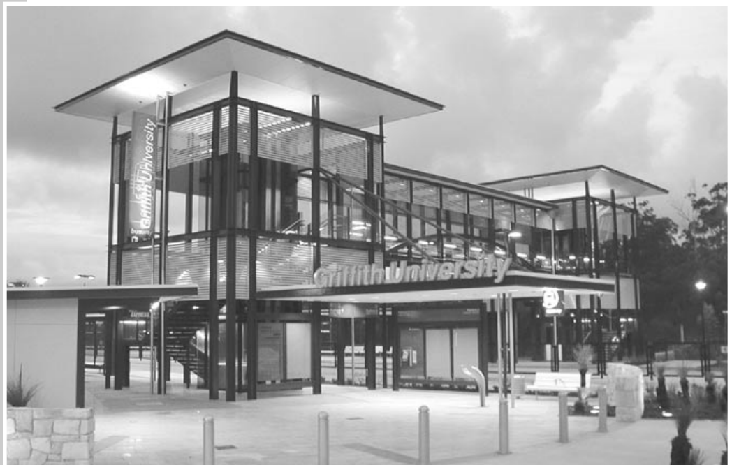
Griffith University Station, SE Busway, Brisbane, Queensland, Australia
